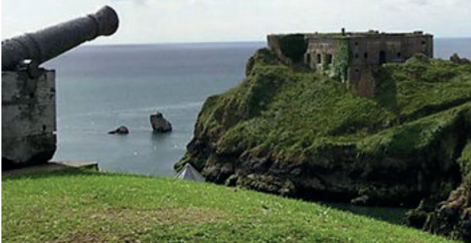
St Catherine's Island & Fort. Copyright George Lloyd Licensed under Creative Commons
