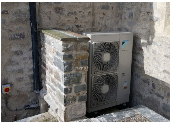
The new air source heating pump - saving both cost and environmental impact.
