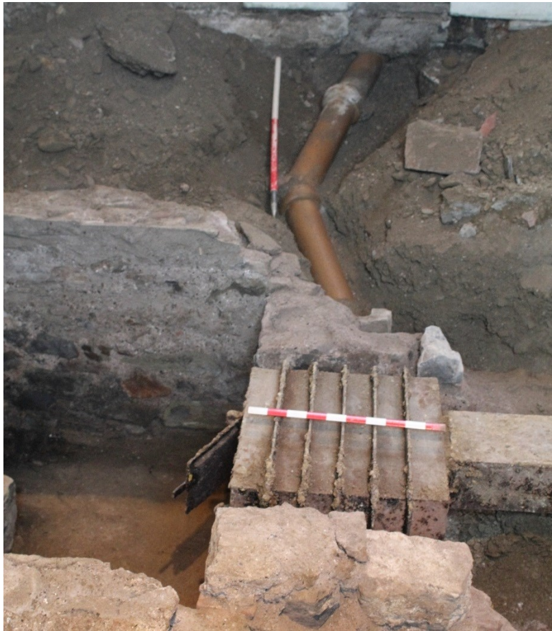
Photo 16: The stove pit and stove, with the northern tuyere coming from the northern wall of the nave and through the base of the small wall to the north of the stove, to provide air for the stove. The near scale is 0.5m long and the far one is 1m long.
