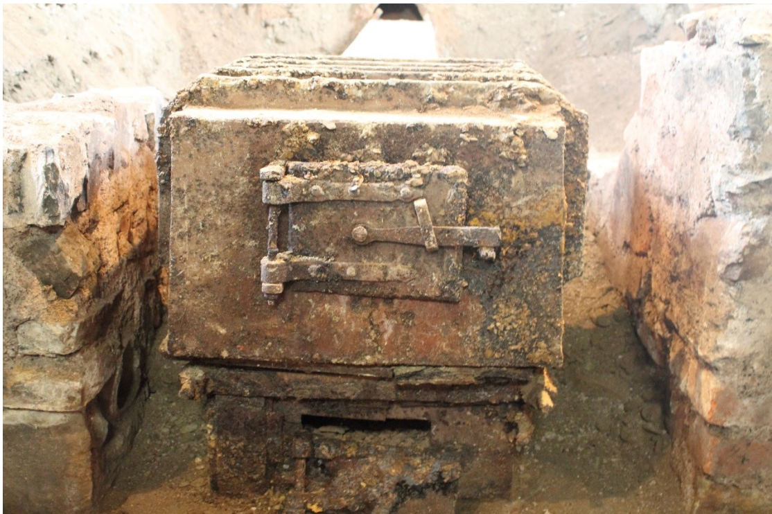
Photo 22: The stove and chimneys, with walls of the pit either side. At the bottom of each wall the end of each tuyere can be seen.
