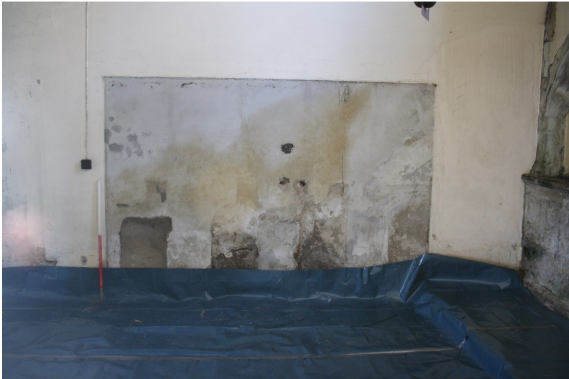
Photo 30: The 'pew ghosts' on the west wall of the north transept, partially covered by subsequent plastering, and surrounded by a large rectangular mark left by a cupboard that was there until recently. Plastic sheeting has been laid down as a base for the new floor. 1m scale.
