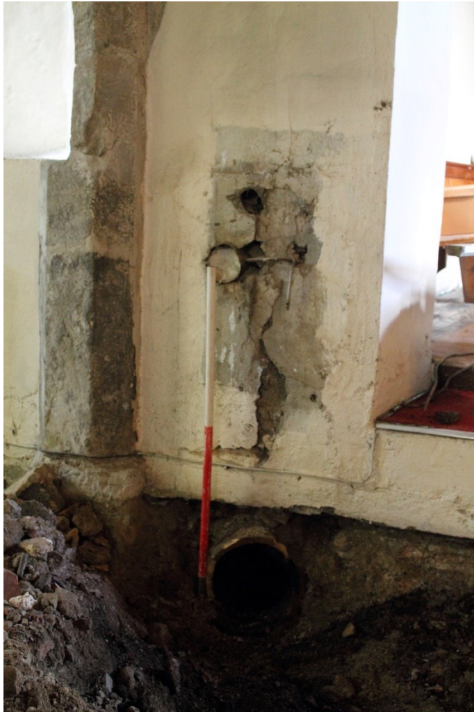
Photo 23: Cross-section through the horizontal ceramic chimney below the previous floor level, and above it in the wall between the north transept and the chancel can be seen components of the vertical chimney embedded in it
