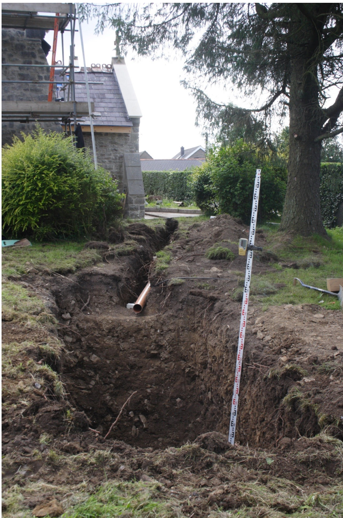
Photo 44: Looking east at the completed excavation of the cess-pit trench and the drainage channels from the porch of the church
