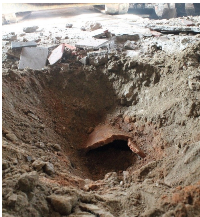
Photo 13: Part of a ceramic pipe was partially drilled through about halfway down the centre aisle of the nave
