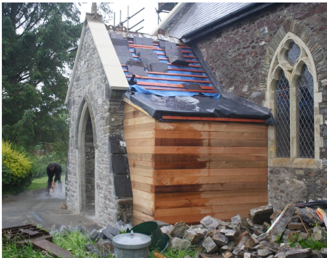
Photo 32: The new toilet building to the east of the porch and the initial cutting of the tarmac for the drainage trench. The stove excavated inside the church is on the grass in the foreground.
