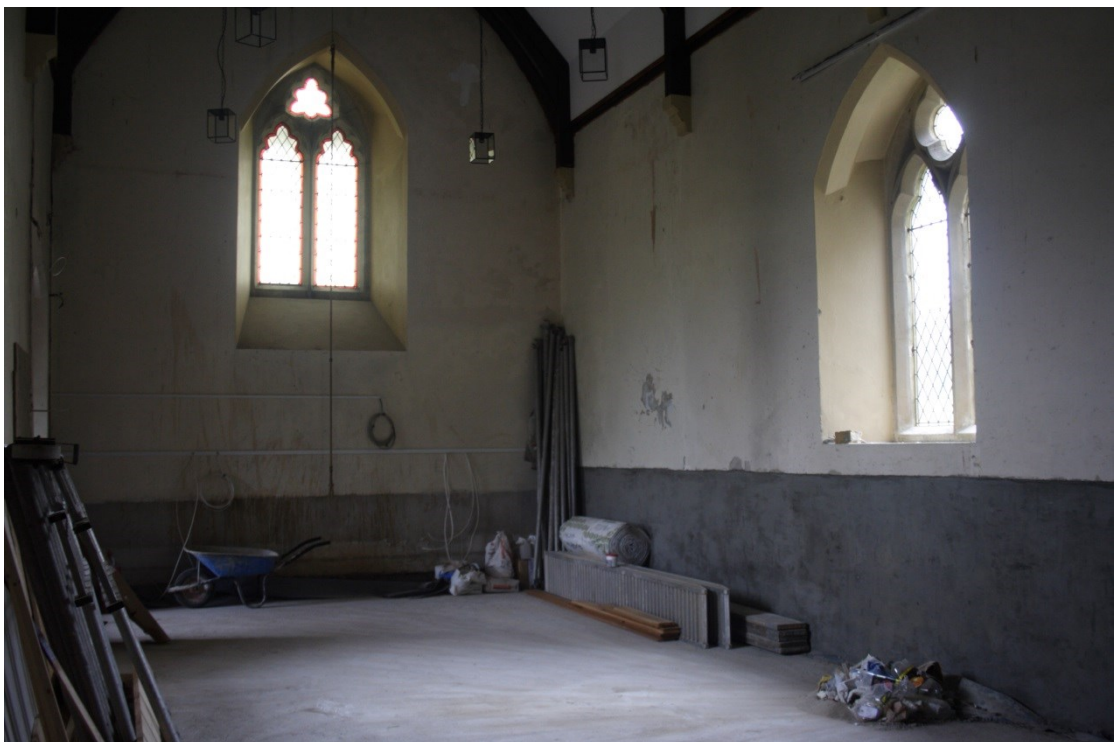
Photo 31: The west end of the nave after insertion of underfloor heating components and concrete flooring, and after plastering of the bases of the walls, covering the pew ghosts.
