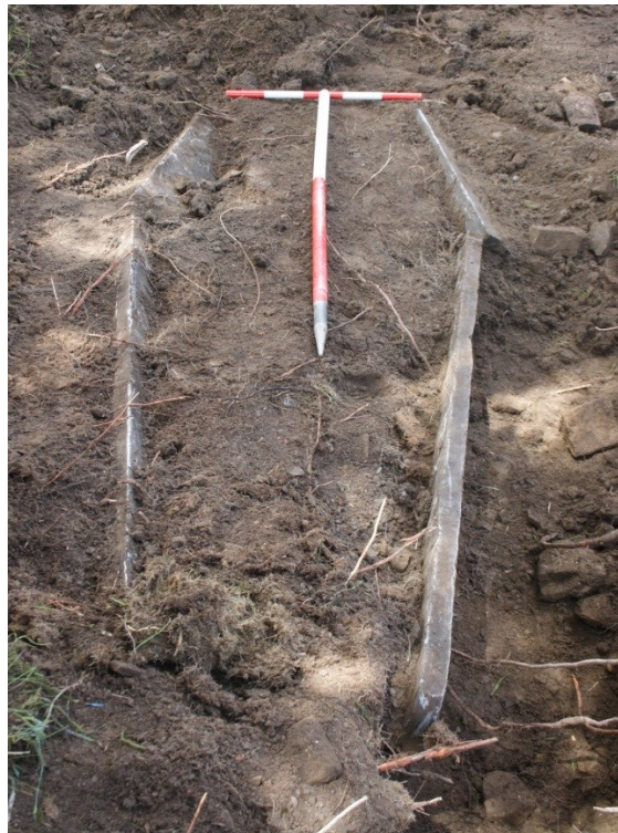
Photo 39: Collapsing kerbstones on either side of a former pathway, discovered just below the topsoil during excavation of the new drainage trench, 0.5m and 1m scales
