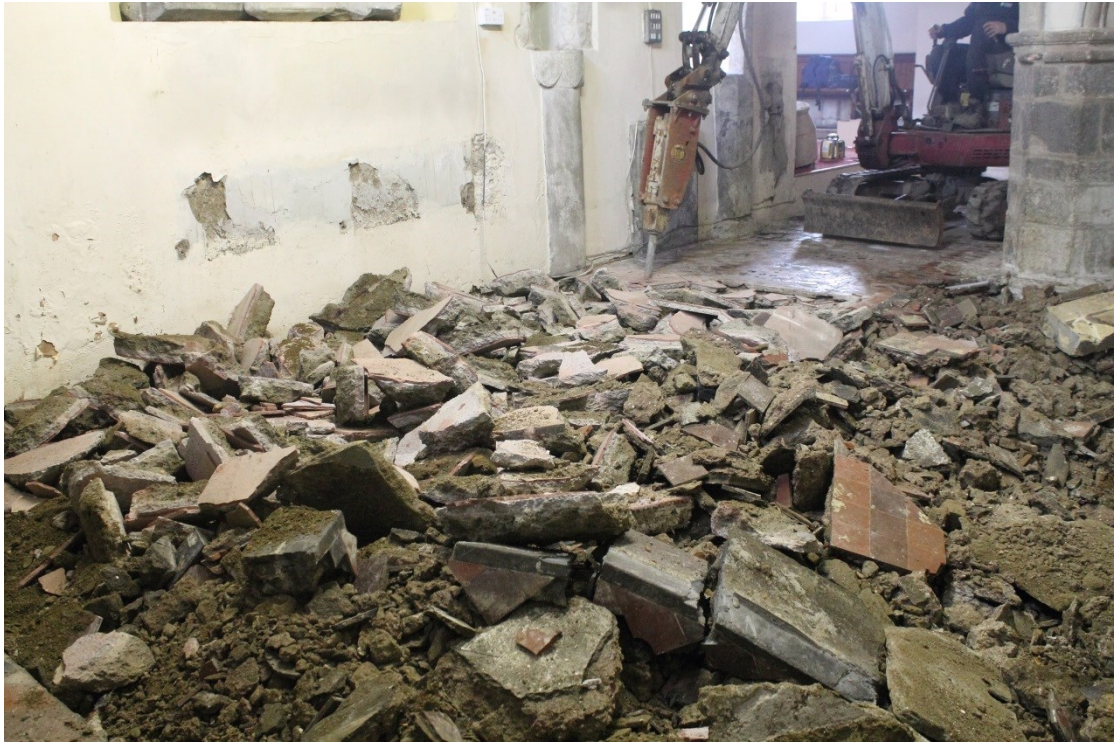
Photo 11: Breaking of the concrete and tile floor on the eastern side of the north transept
