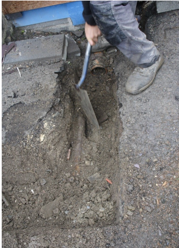
Photo 33: An old drainage pipe is revealed during excavation of a new drainage trench, just south of the new toilet building. The end of the new drainage pipe can also be seen, already put in place when the toilet was built.
