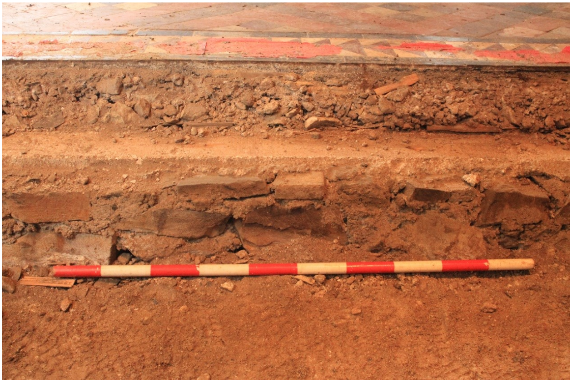
Photo 7: A short section of the dwarf wall foundations supporting the Victorian floor above, 1m scale
