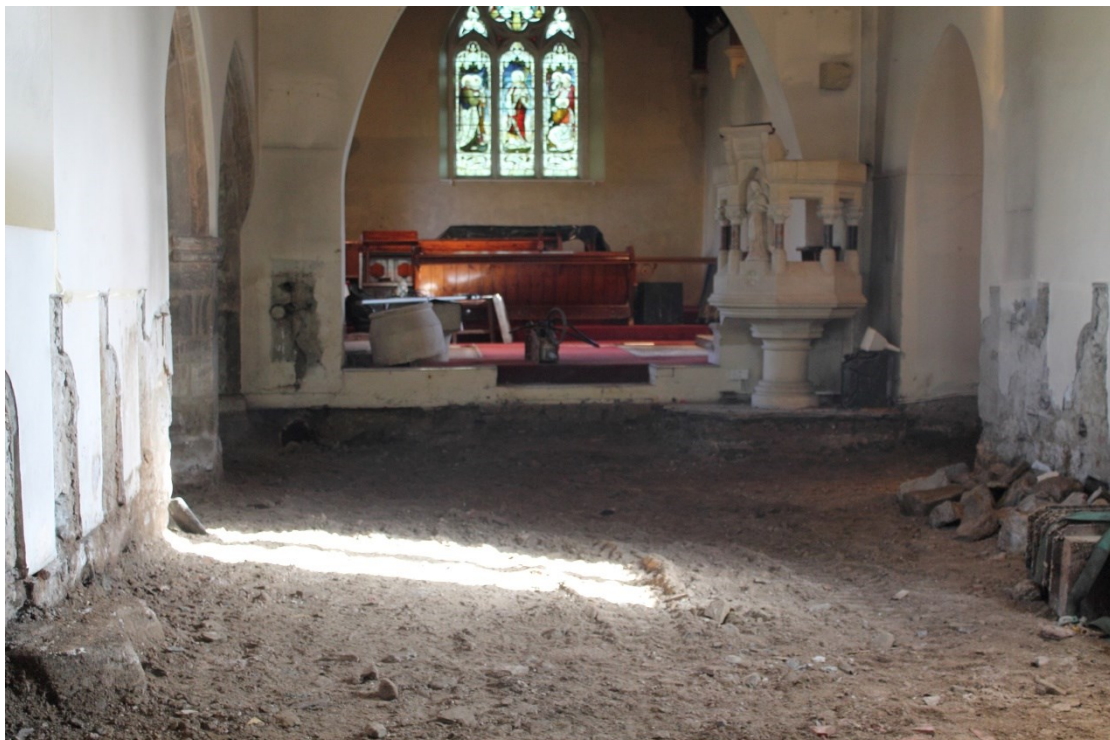
Photo 27: The east end of the nave after completion of excavation of the rubble layer beneath the old wooden floor to the required depth of 0.3m
