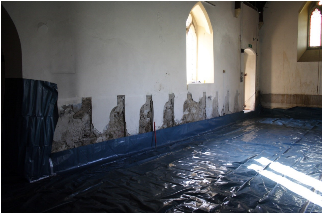
Photo 29: The south side of the nave after the laying down of plastic sheeting as a base for the new floor. 'Pew ghosts' line the wall, with a 1m scale.
