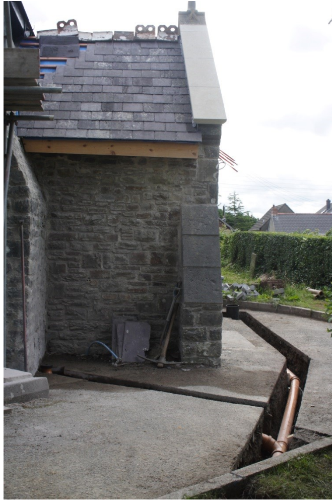
Photo 36: The drainage trenches from the sink and toilet after excavation and insertion of plastic pipe, in the area of the tarmac path outside the porch
