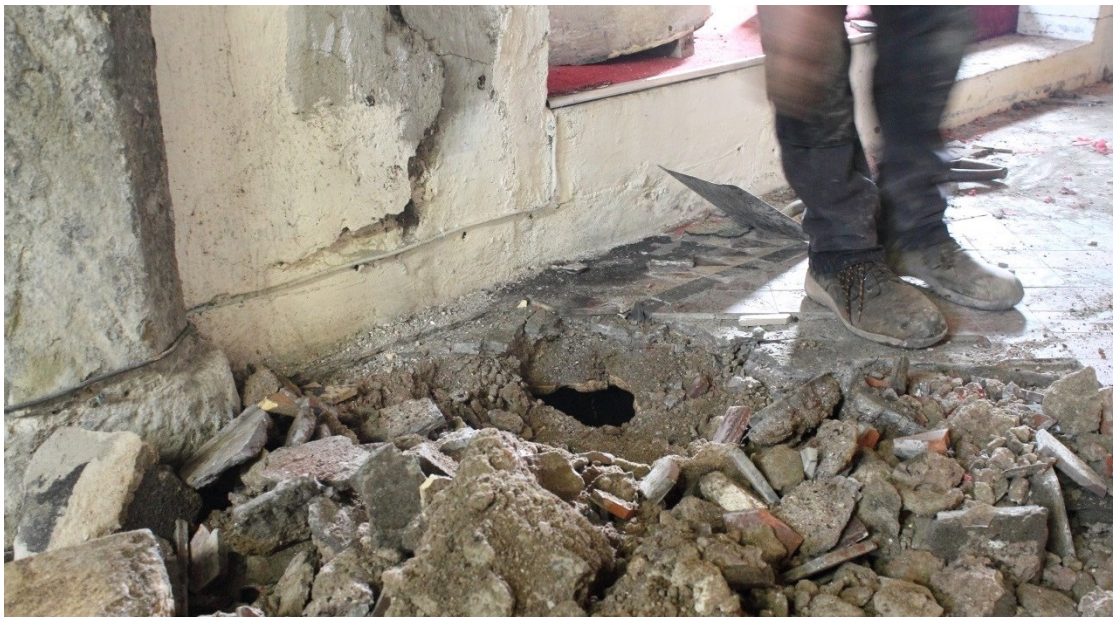
Photo 12: A small void shows where part of a ceramic pipe was partially drilled through on the corner between the north transept and the chancel
