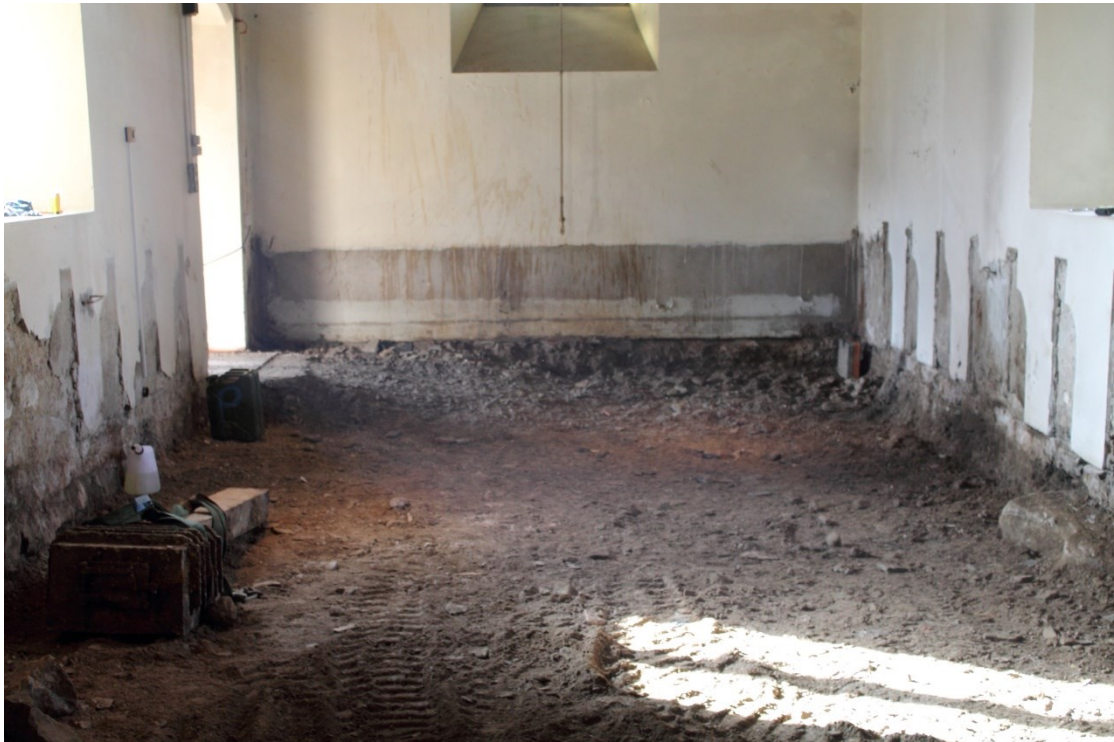
Photo 28: The west end of the nave after completion of excavation of the rubble layer beneath the old wooden floor to the required depth of 0.3m
