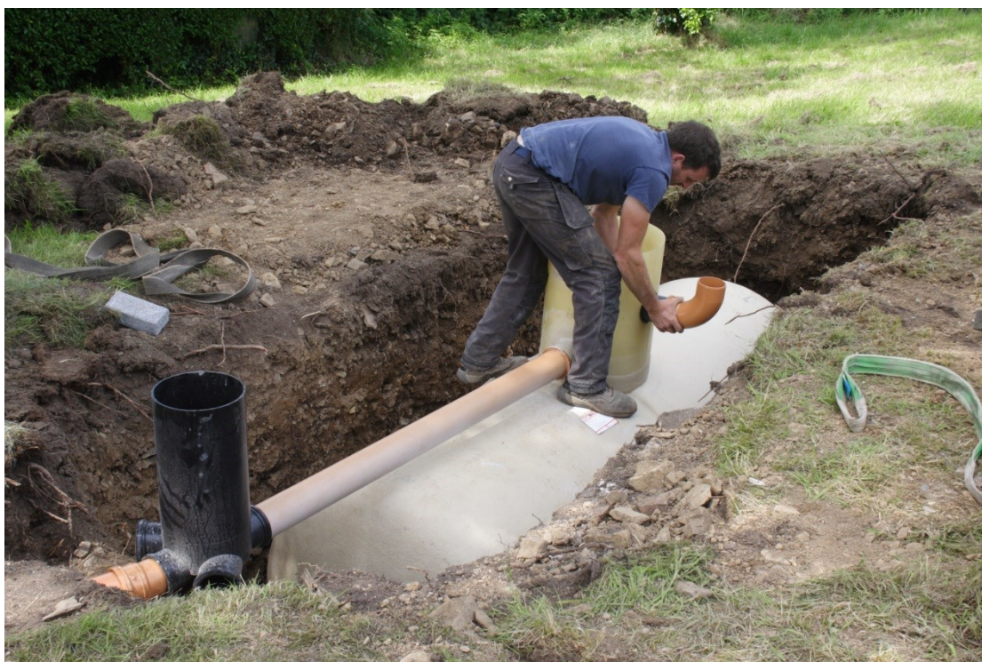
Photo 46: The new cess-pit tank after positioning in its trench
